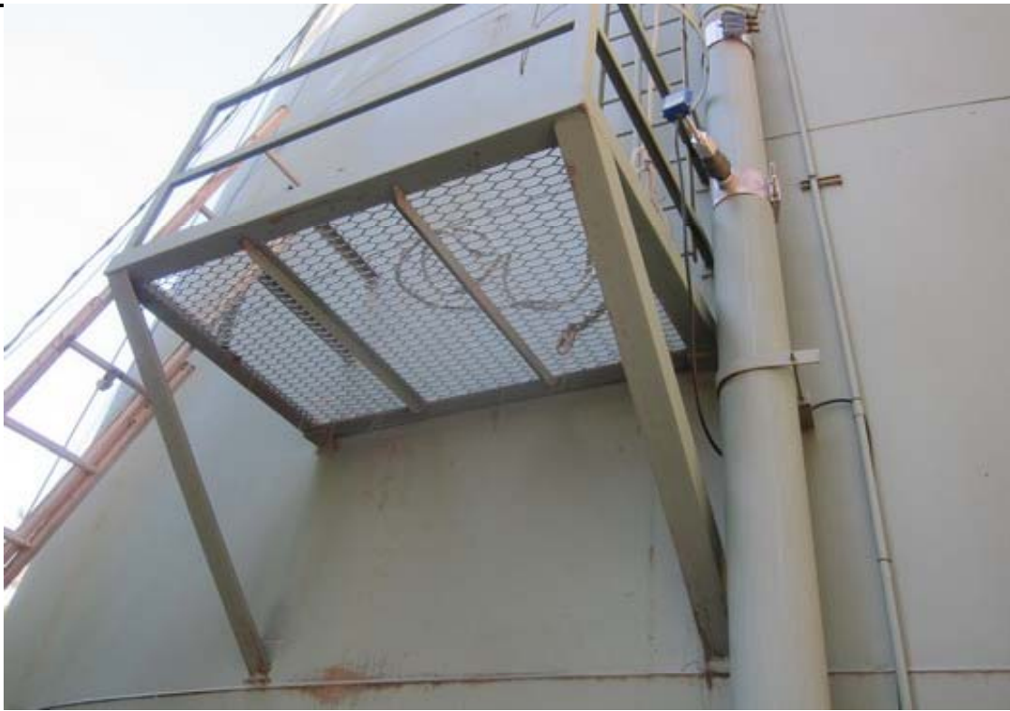
MG#2 Existing ladder platform
