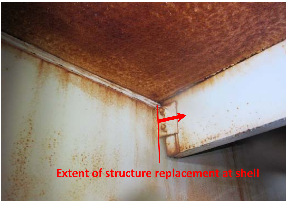
MG#1 existing rafter and shell clip and extent of roof structure replacement at the shell.
