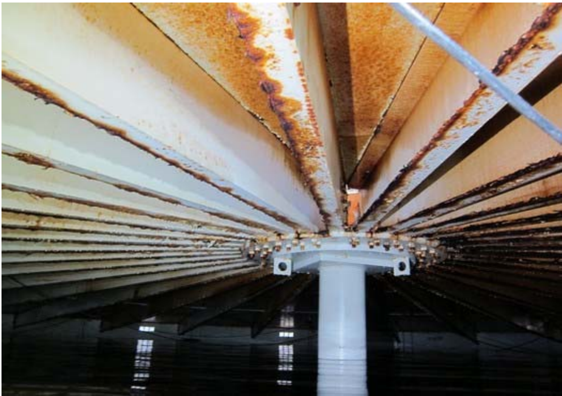
MG #2 existing interior center support and rafters.
