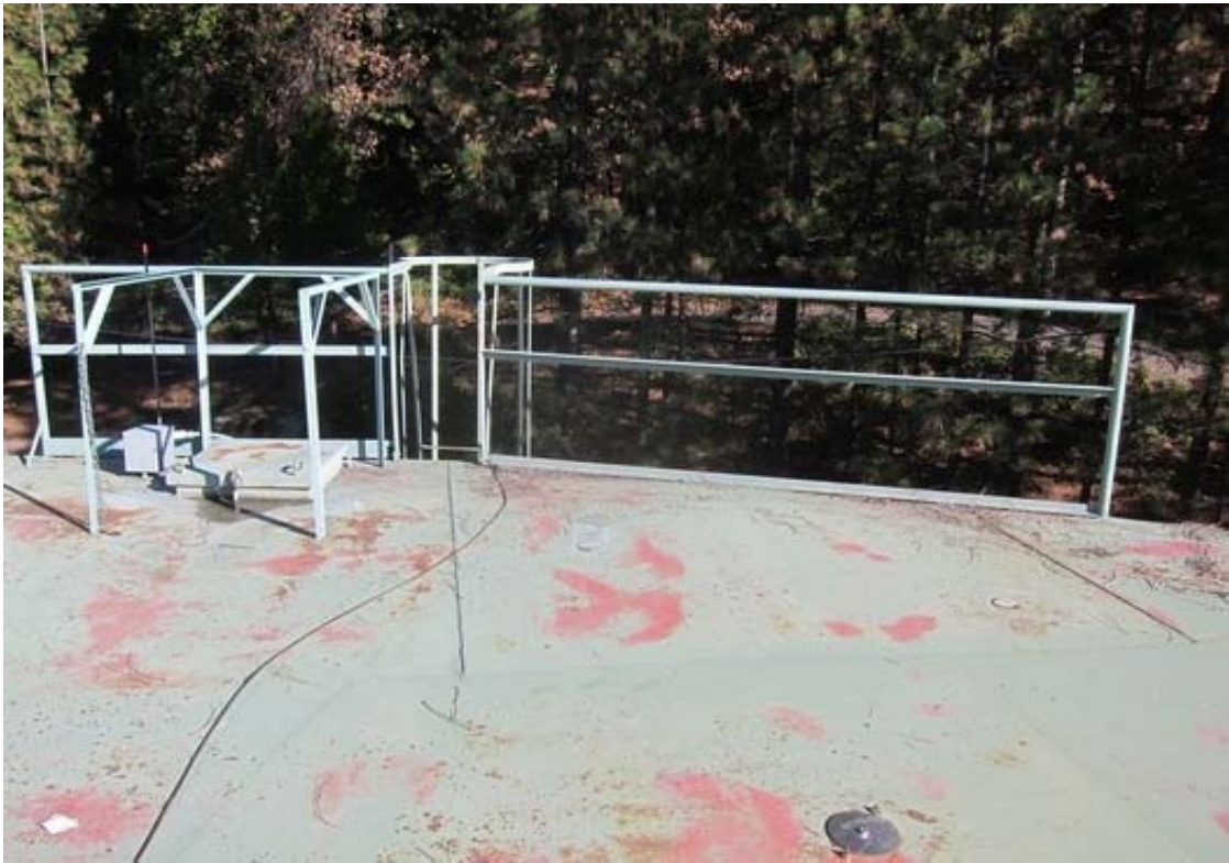
MG#1. Existing roof hatch area.
