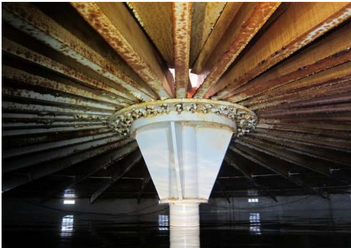
MG #1 existing interior center support and rafters.
