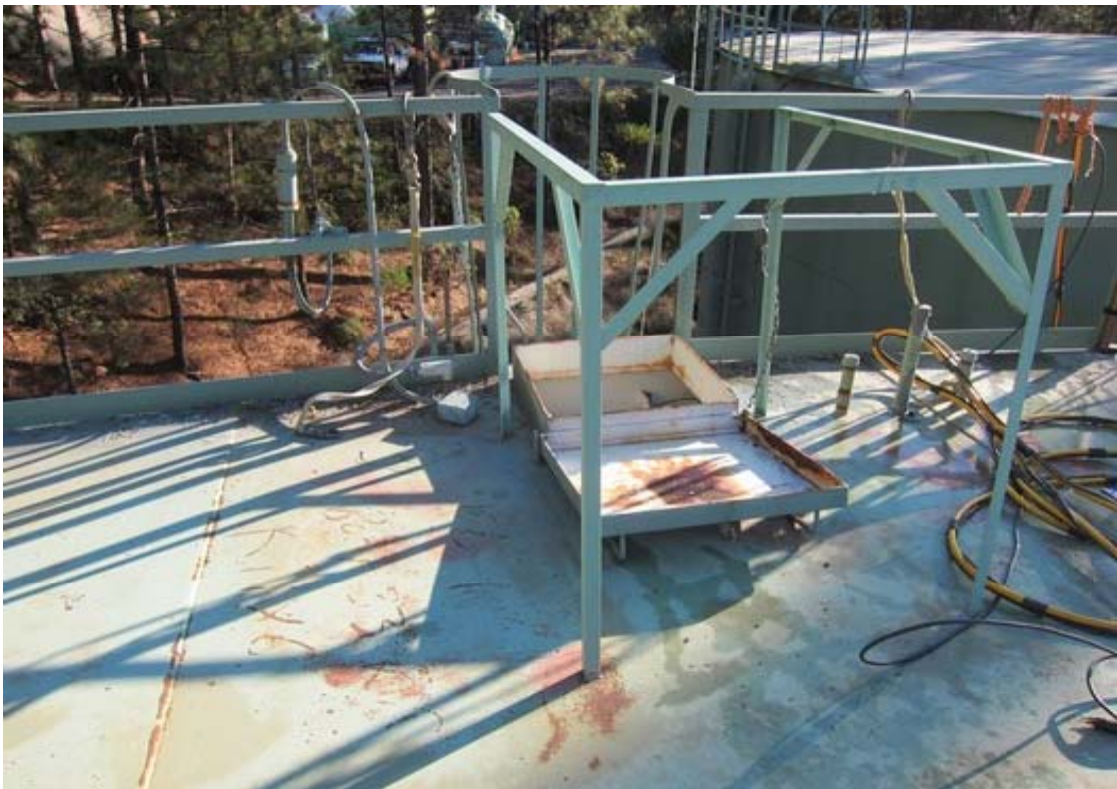
MG#2 Existing roof hatch, guardrail and appurtenances.
