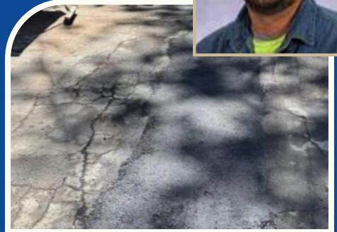
All paving repairs were completed.
