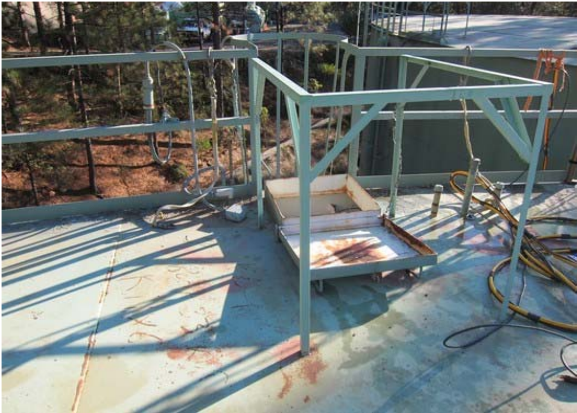
MG#2 Existing roof hatch, guardrail and appurtenances.
