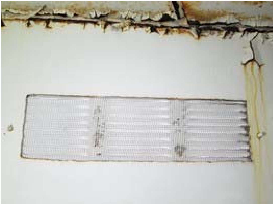
View of typical existing shell vent. Cover plates are to be installed as part of the Work.
