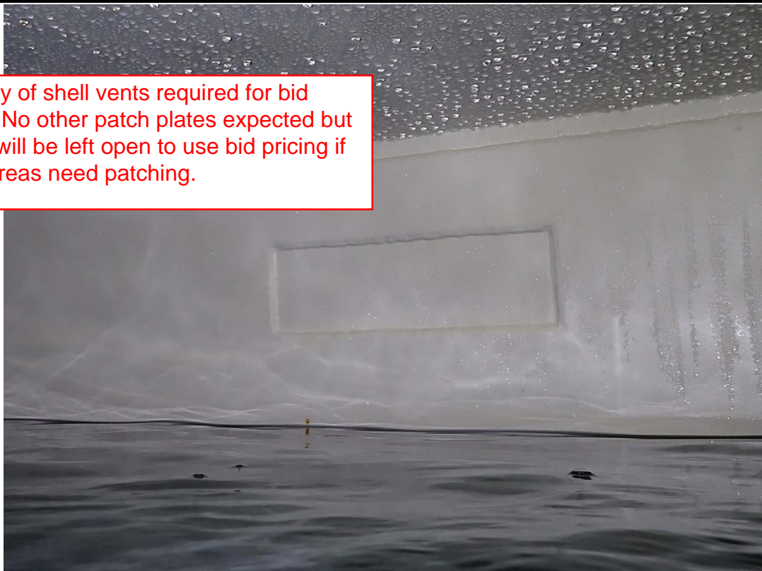
View of acceptable shell vent closure.
