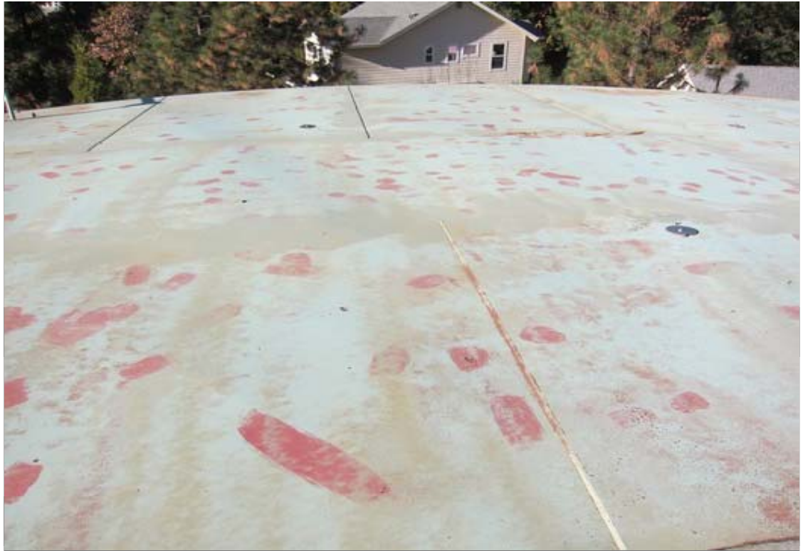
This view indicates the overall condition of the roof. The roof plate (steel) is in good condition but coatings are in poor condition.
