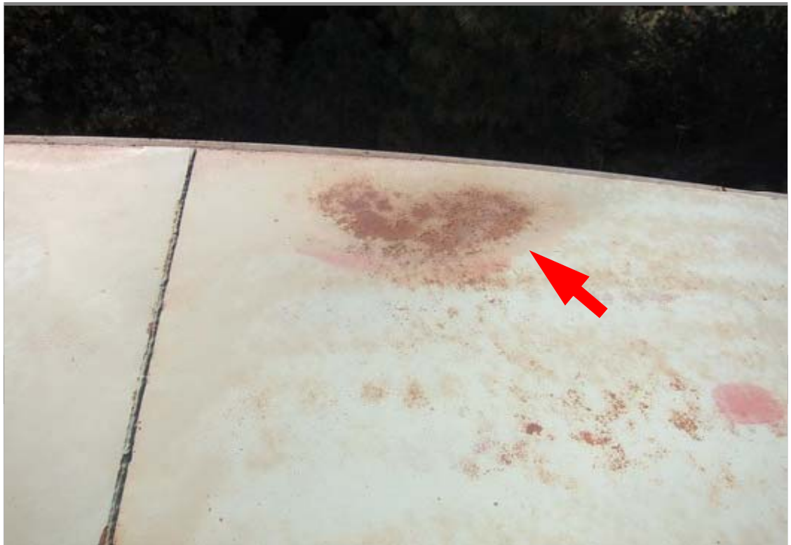
Close view of a ponding area with corrosion. Submersed exterior coatings pose a maintenance challenge.
