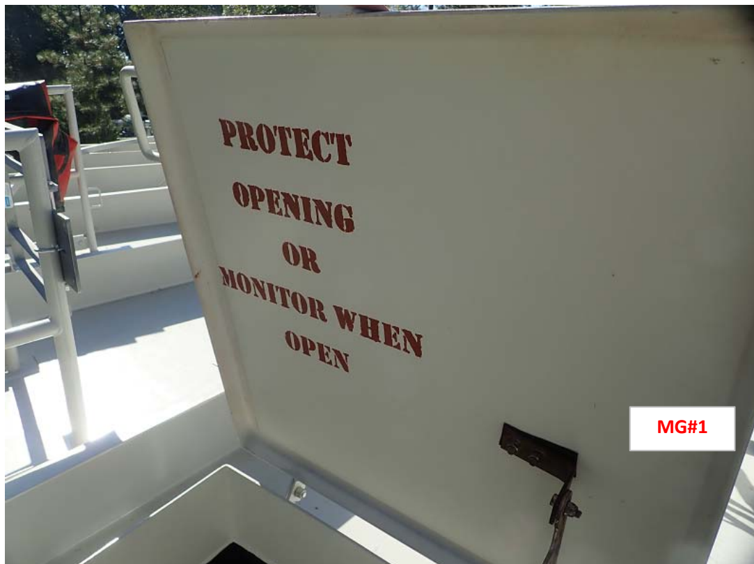
Signage required on new roof hatch.
