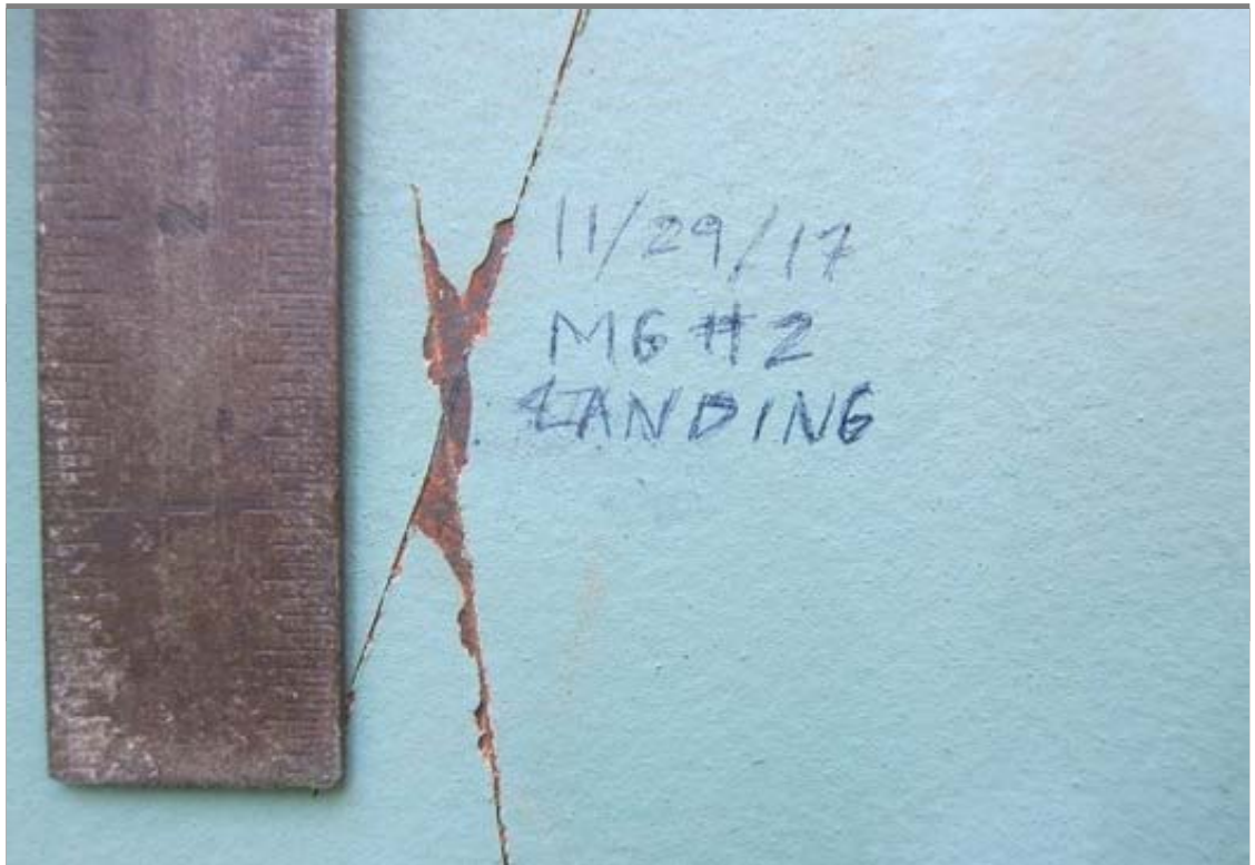
Adhesion was evaluated with a cross cut tape test and found to be 2A-3A. This location was on the exterior shell at the mid platform.
