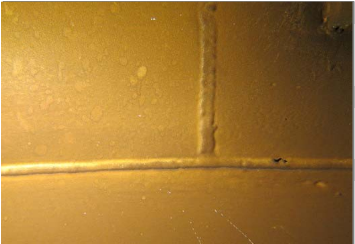
Interior shell in the submersion zone. This view shows a junction between a horizontal and vertical shell joint. The interior shell steel appears to be in good condition overall.
