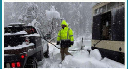
Garrett Collum refueling the Shadybrook Generators
