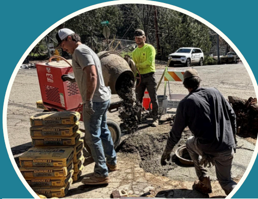
JB Excavation repairs manhole at Marquis and Golf Club
