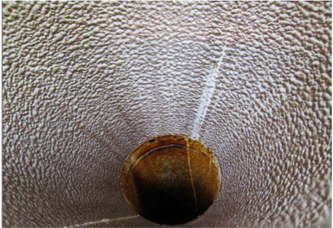
Interior of the overflow weir.
