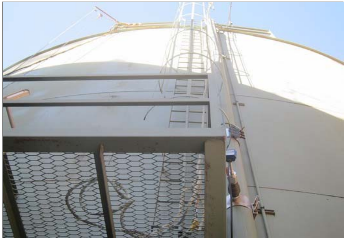
This view from the ground shows the platform, exterior ladder and cage. No significant corrosion is present. The climber safety rail has been painted.
