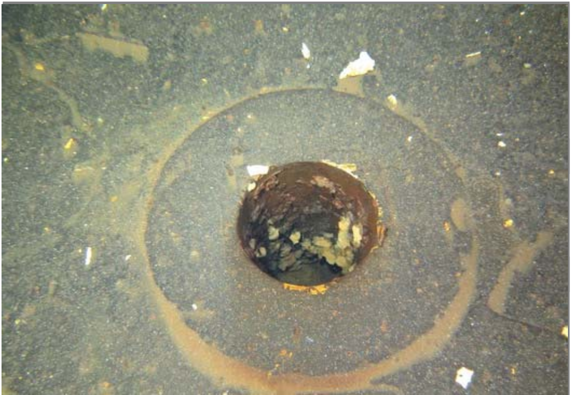
An additional view showing the interior of the drain.
