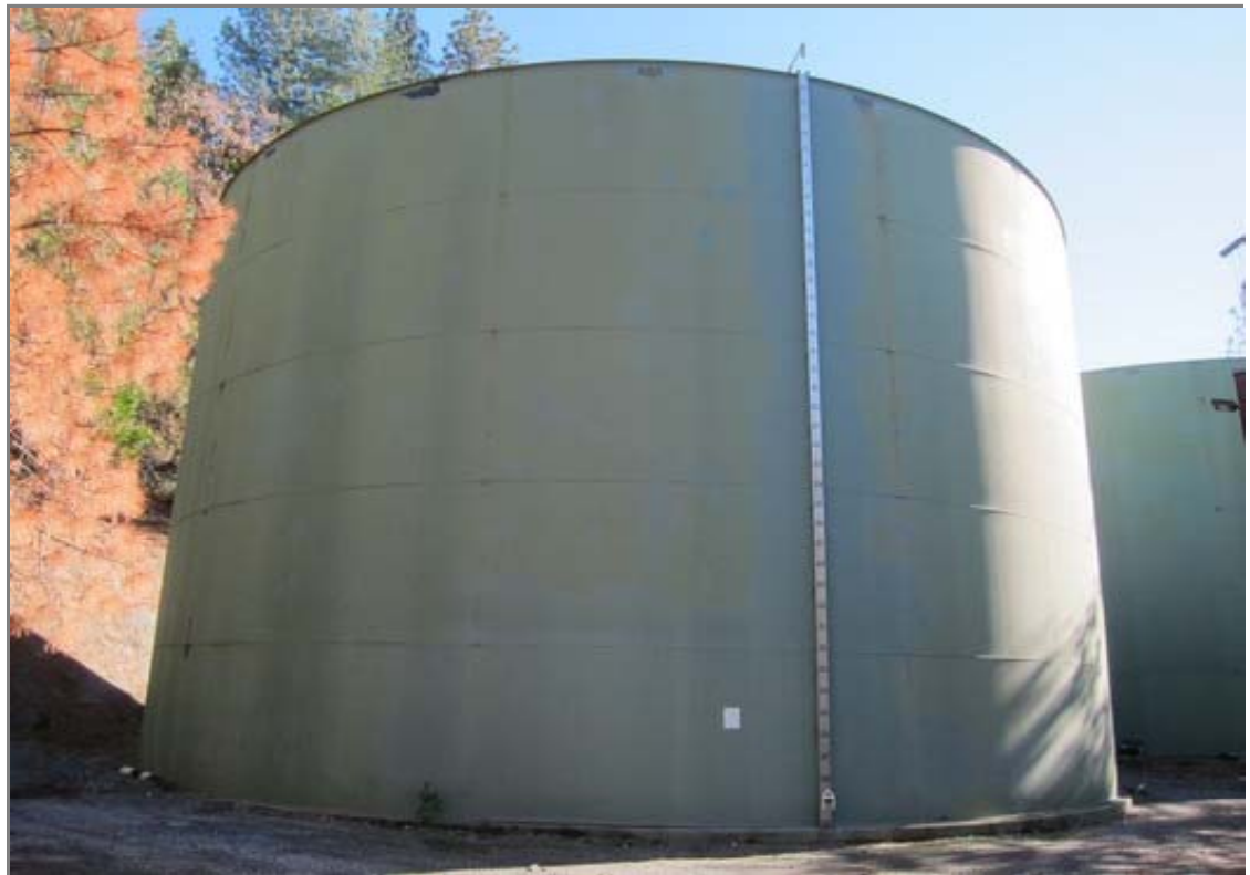
Overall view of the MG #2 Tank.
