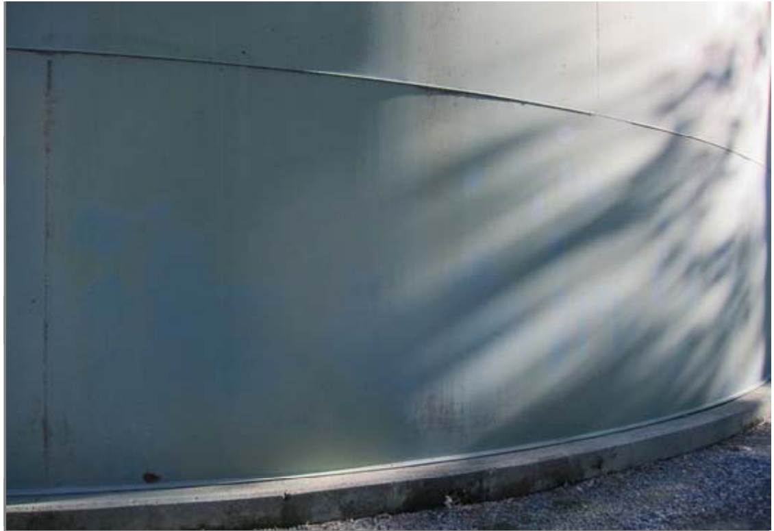
Lower shell and concrete footing. No significant corrosion points were identified.
