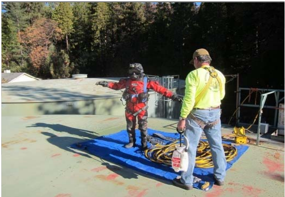
Diver and equipment are disinfected with the chlorine solution just prior to entry. This procedure is pursuant to AWWA disinfection standards for potable water diving.
