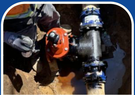
Tie-in for the Manzanita Ct. waterline upsizing.
