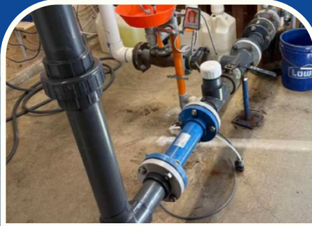
The corroded pipe at well #2 was replaced.
