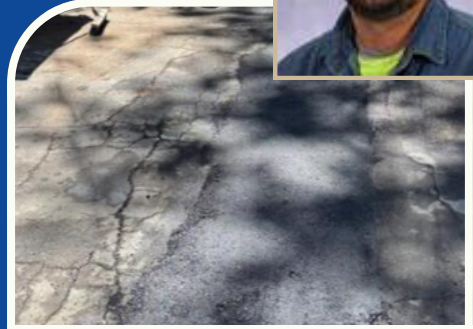
All paving repairs were completed.
