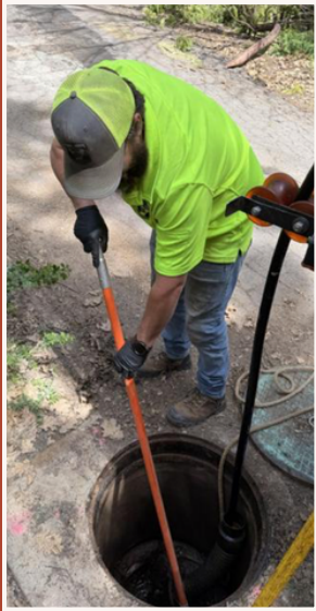
Routine sewer jetting & manhole inspections work.
