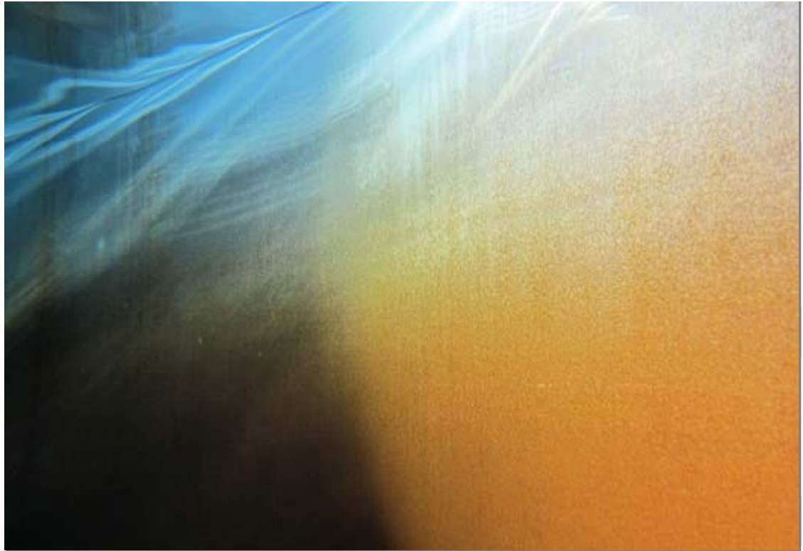
The photo above shows the interior shell just below the water surface (submersion zone). The rust color on the shell is staining.
