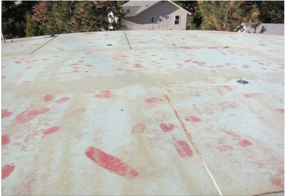
This view indicates the overall condition of the roof. The roof plate (steel) is in good condition but coatings are in poor condition.
