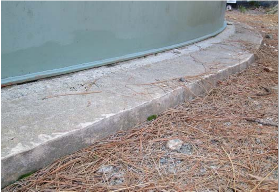
Lower shell and concrete footing. No significant corrosion points were identified. Some significant cracks and concrete corrosion are present in the concrete.
