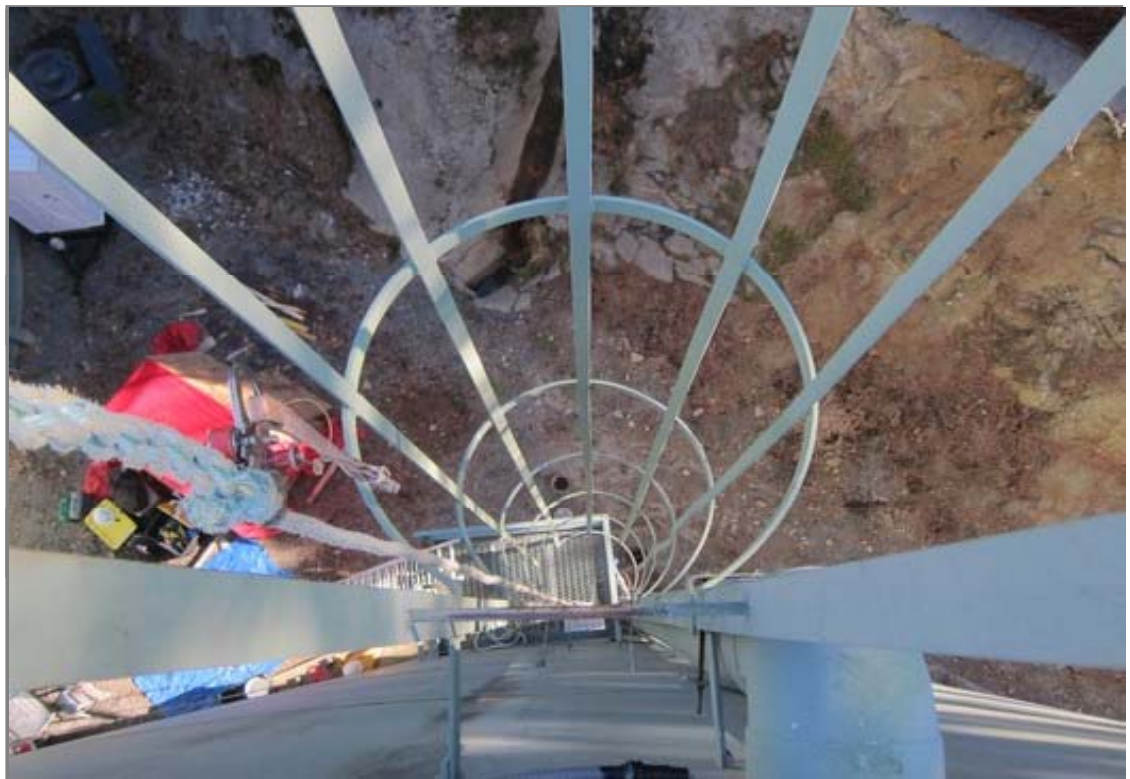
This view from the top of the exterior ladder and cage. No significant corrosion is present. The rung width is 15".
