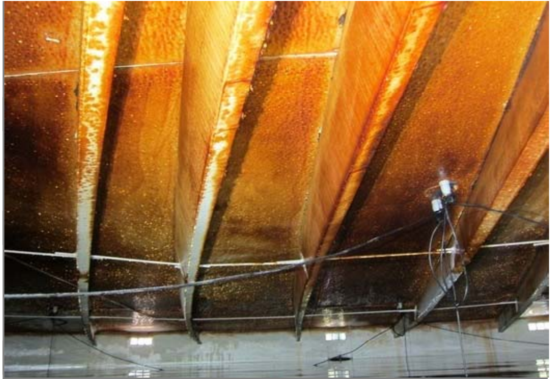
Interior roof plate, rafters and bracing. Typical broad view. Approximately 20 of the rafters have "rolled" which could be due to a past over-stress condition such as lateral loads from seismic sloshing or heavy snow load or other types.
