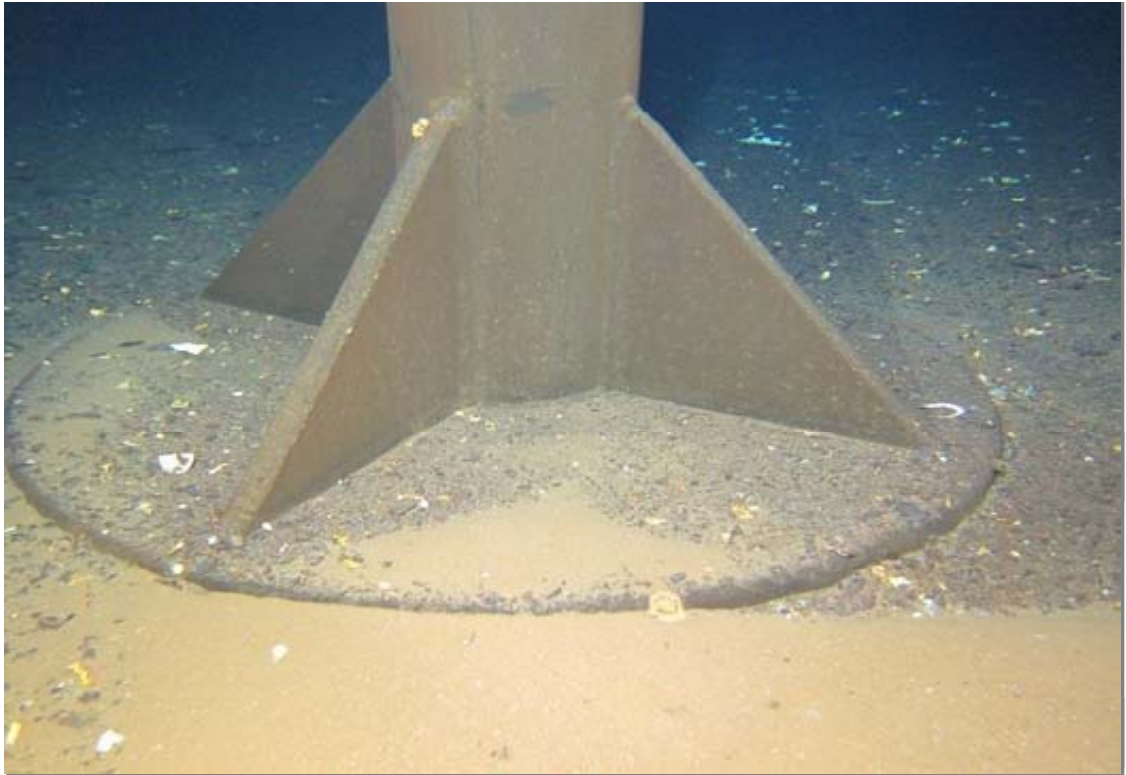
This view shows the column base plate and adjacent bottom plate. Coatings are in good condition overall on the column and base plate. Approximately 10 corrosion points are present along with some associated metal loss.
