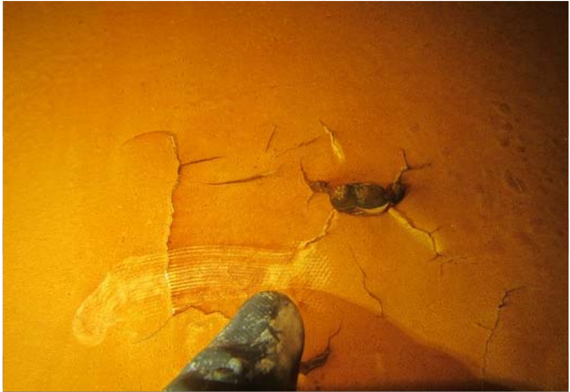
Interior shell in the submersion zone. This view shows one of approximately 20 areas of damaged coating in the lower shell. The coatings have cracked and corrosion is present.
