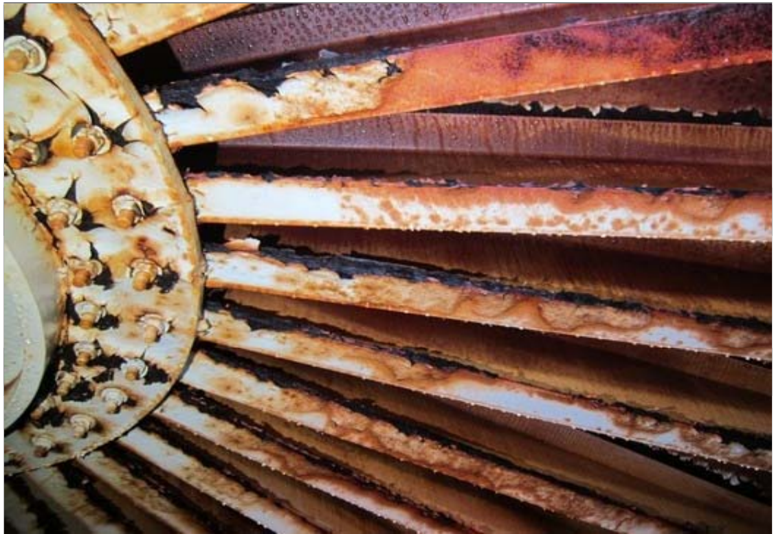
Close view of the center support and rafters. Coating failure and associated corrosion are visible.
