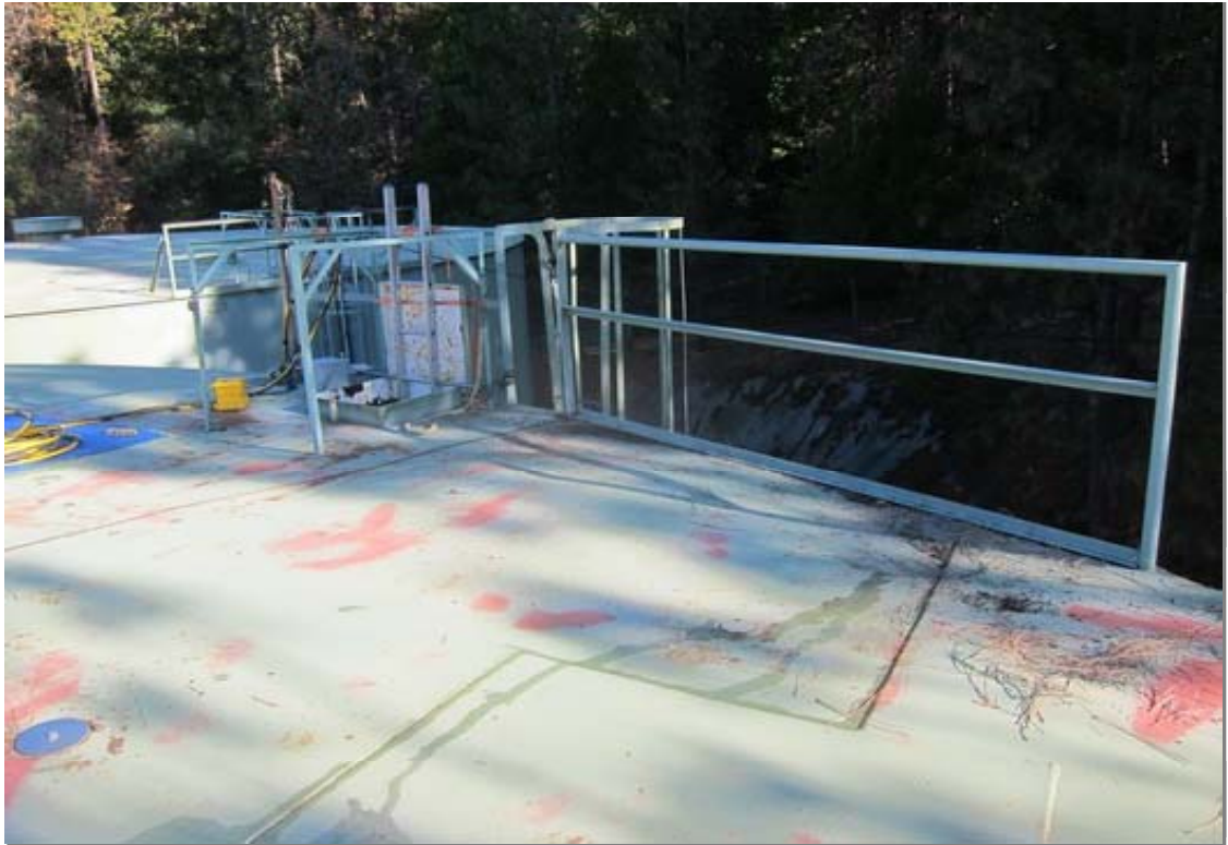
The photo above shows the roof hatch area with guardrail.
