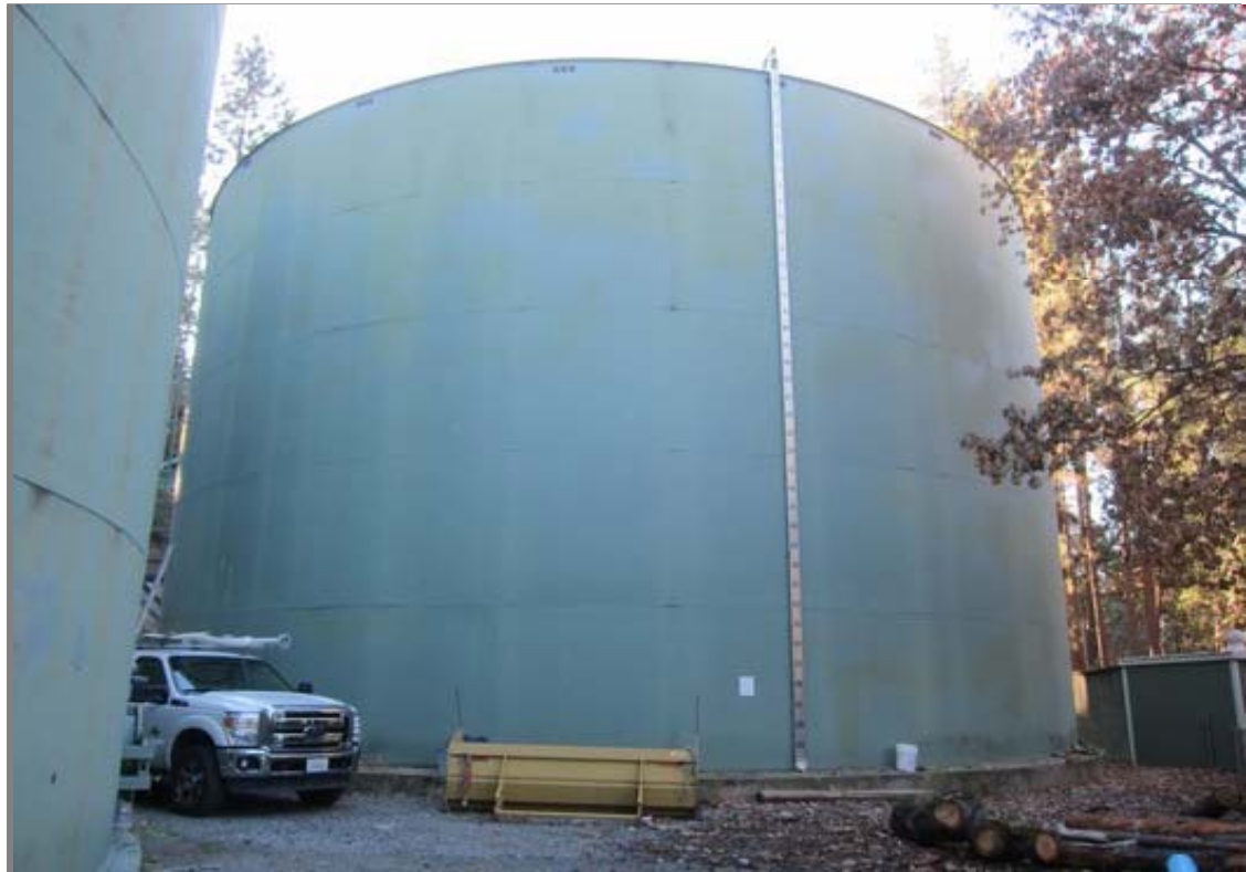
Overall view of the MG#1 Tank.
