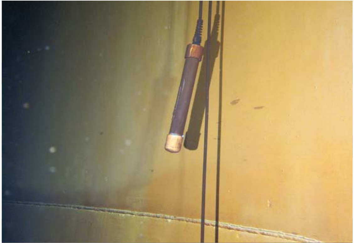
This appears to be a cathodic protection system reference cell.
