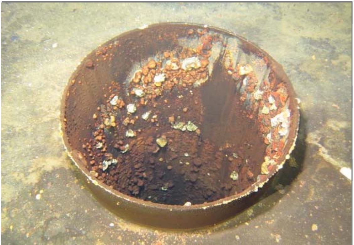
Additional view of the outlet.
