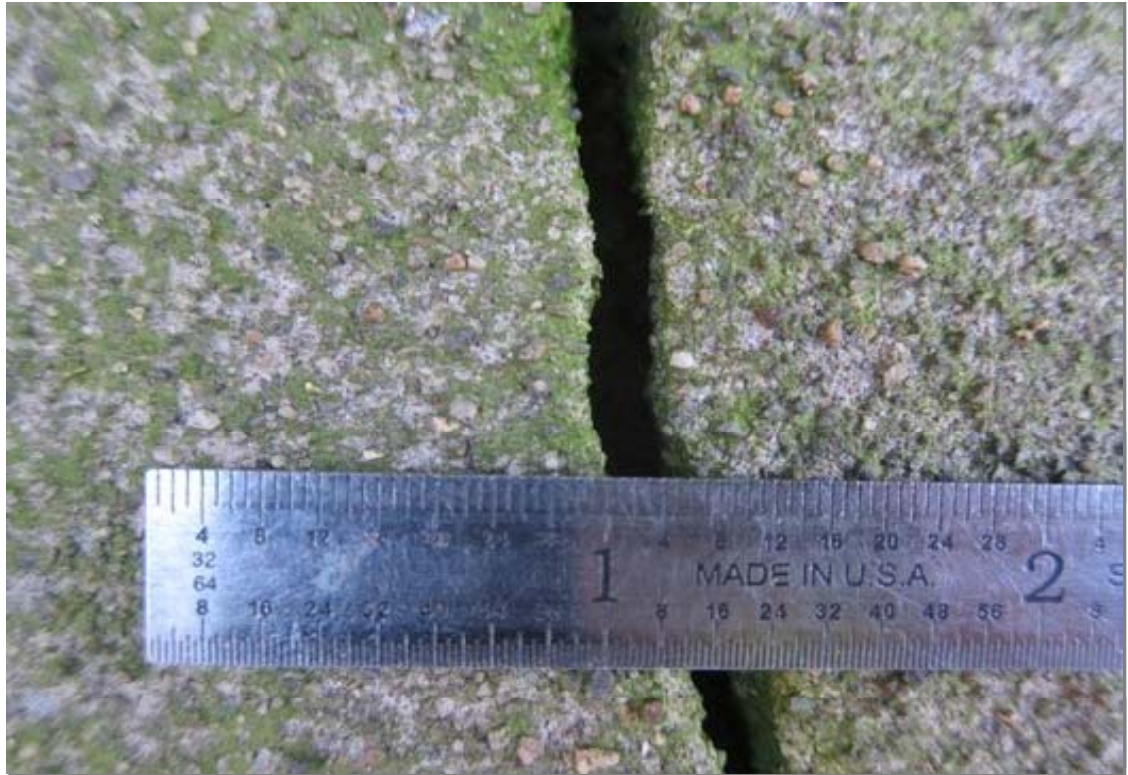
This view of a typical crack in the concrete footing shows approximately 3/16 width"
