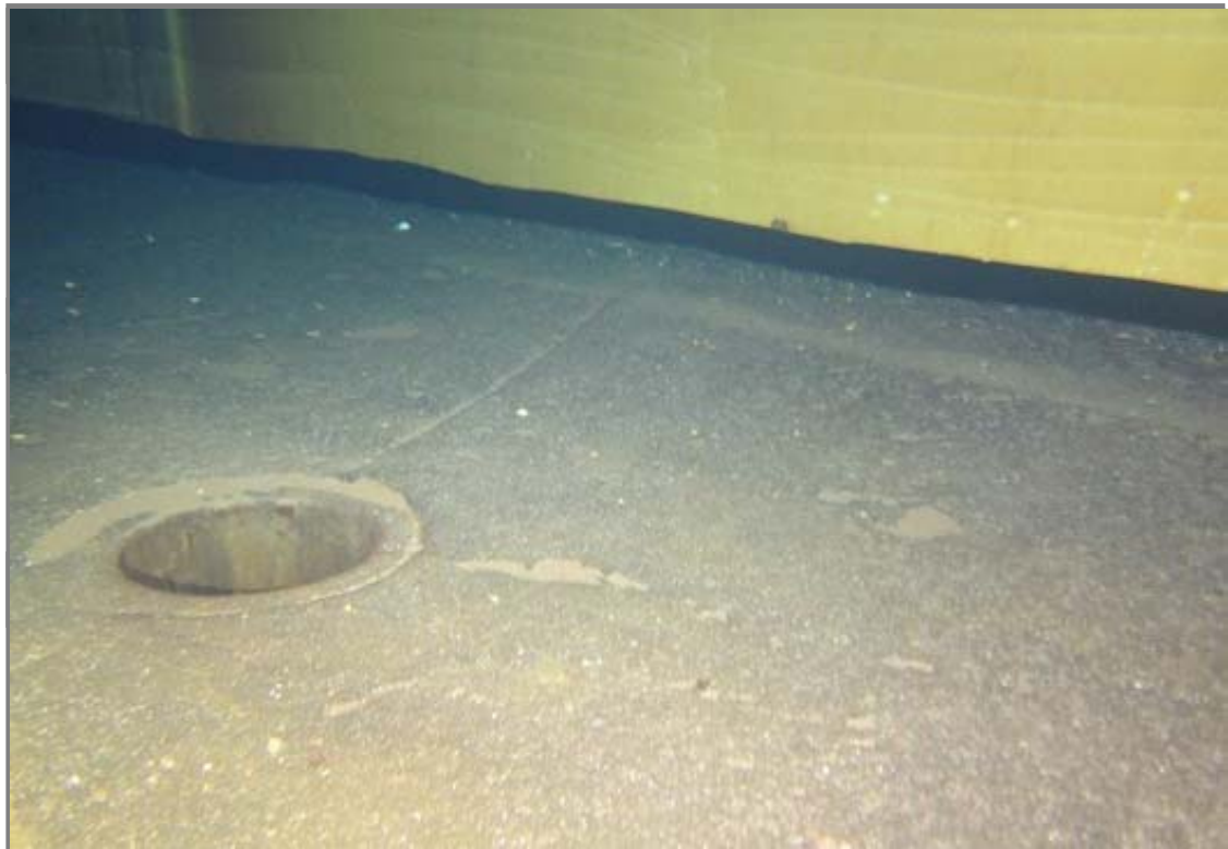
Interior view of the drain. The drain is approximately 4 ft. from the shell.
