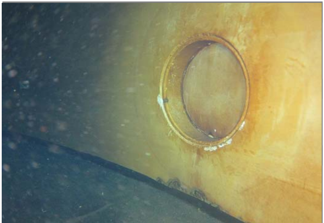
Round shell manway as viewed from the interior.
