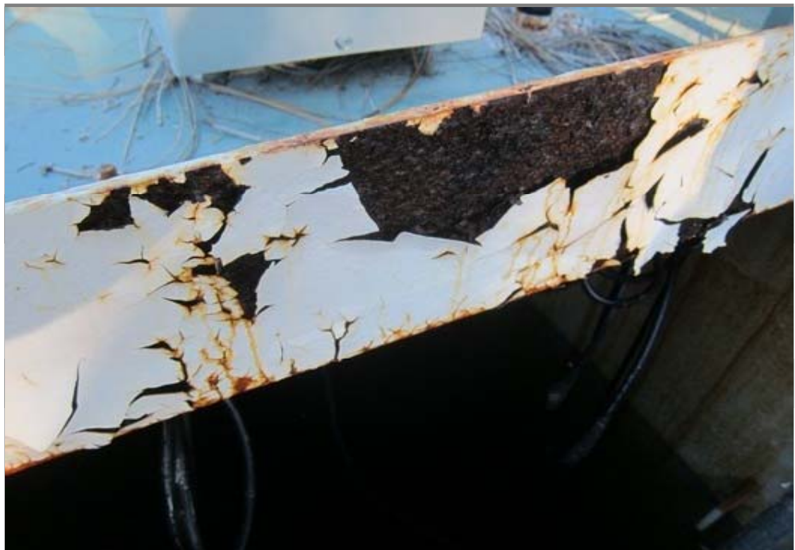
Corrosion and roughening on the interior side of the roof hatch.
