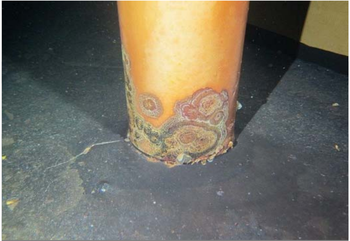
Overflow riser pipe with corrosion near the bottom.
