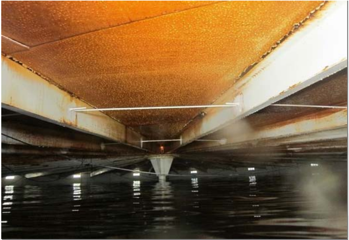
Roof as viewed from the water surface.
