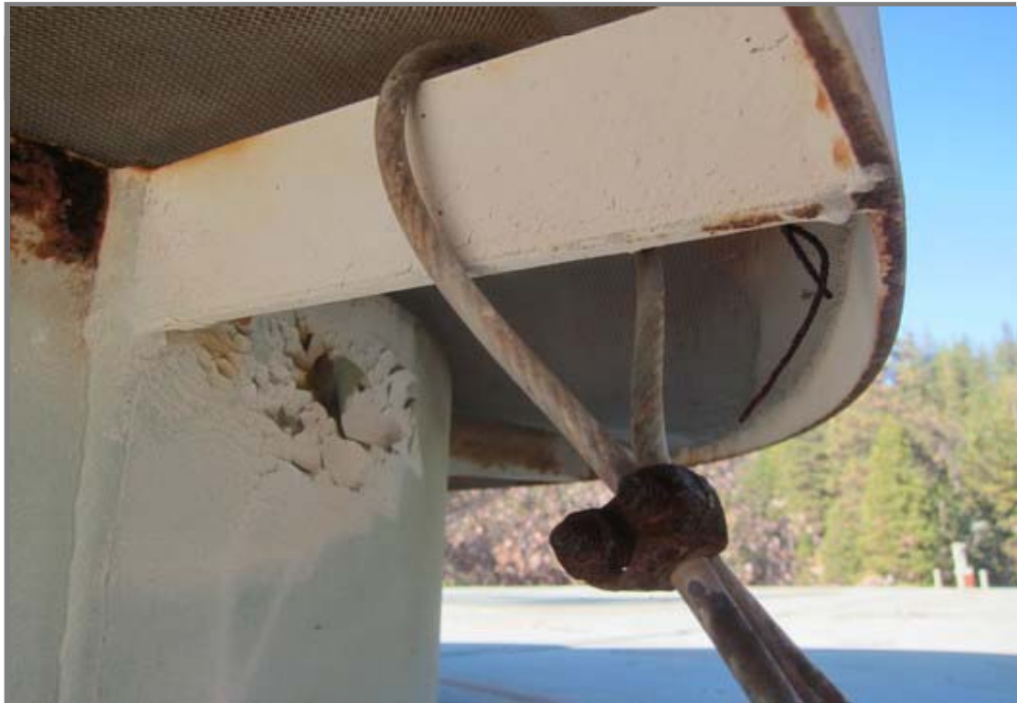
This view of the underside of the vent hood shows that the screen is in good condition. Corrosion is present on the riser but the screen appeared to be bug proof. It appears that this cable may be intended for fall protection but it appears to be inadequate.
