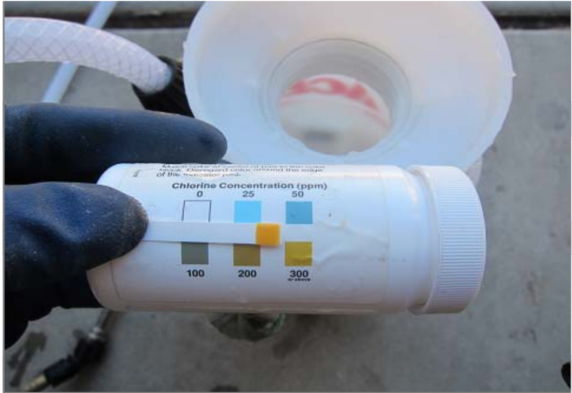
The disinfecting solution is tested to verify that it exceeds the 200 ppm free chlorine concentration level.
