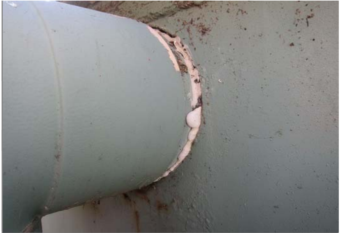
High inlet at shell penetration which is just below the roof. The inlet is PVC.
