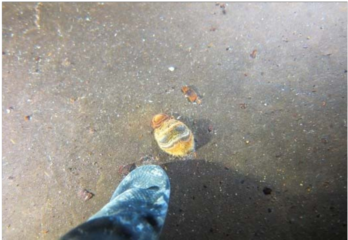
This view shows a rust nodule on the bottom with the diver's finger also visible. This nodule is representative of the scattered corrosion points found on the bottom.
