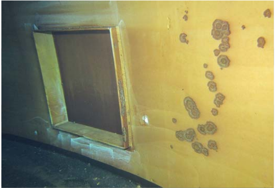
Interior view of the rectangular shell manway.
