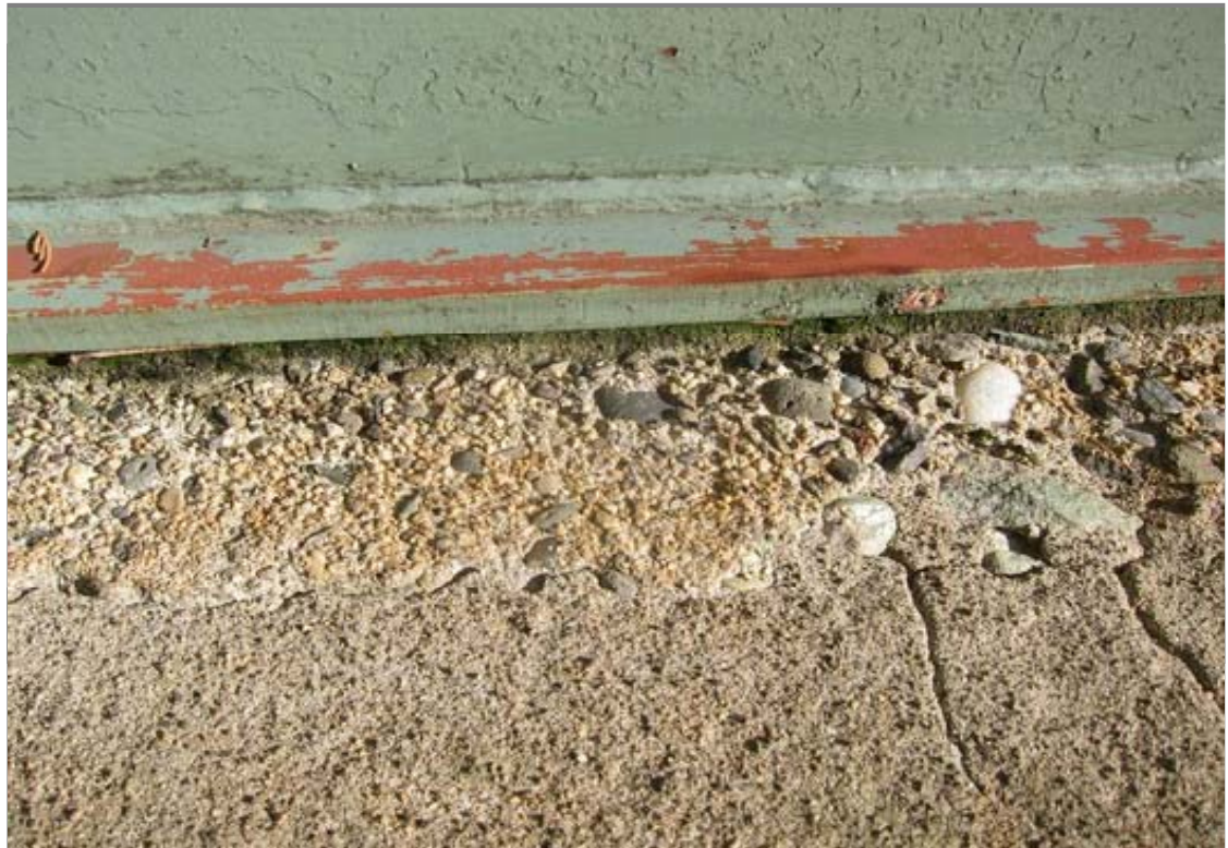
Corrosion of the concrete on the southern side of the tank. Cementitious material is lost but not aggregate. The 5/8" annular ring is visible extending outward from the bottom.
