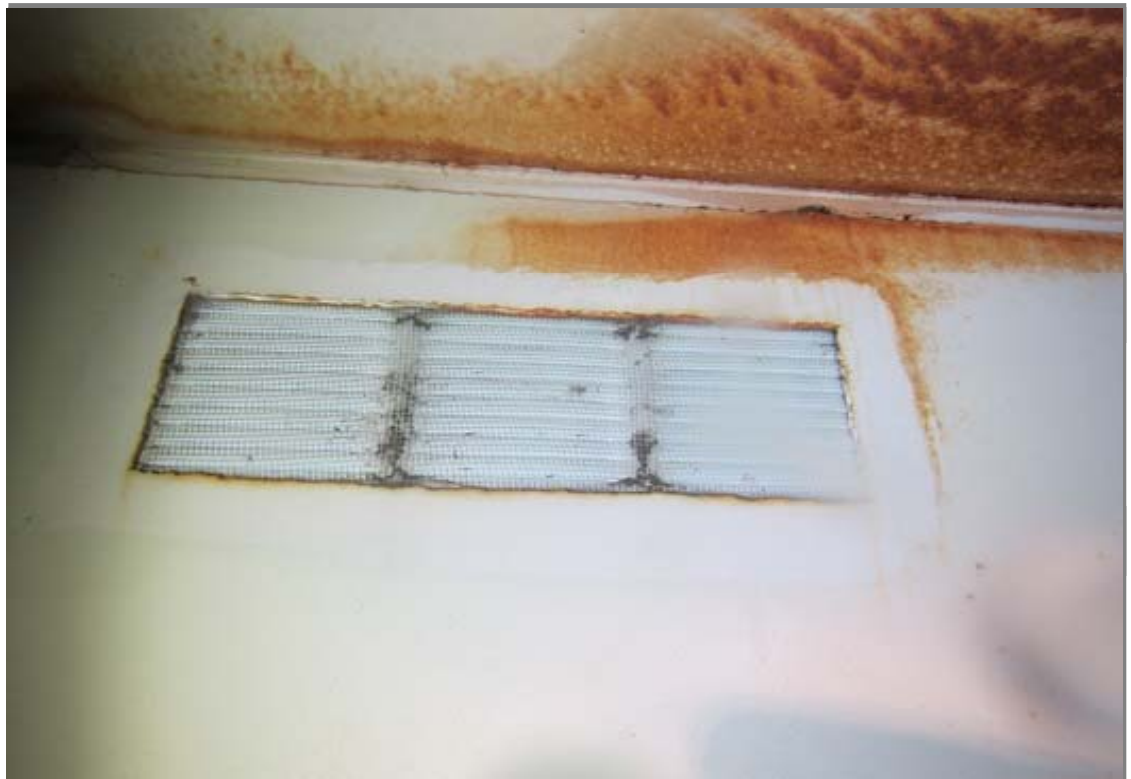
This is a close view of the upper shell showing one of the numerous shell vents.
