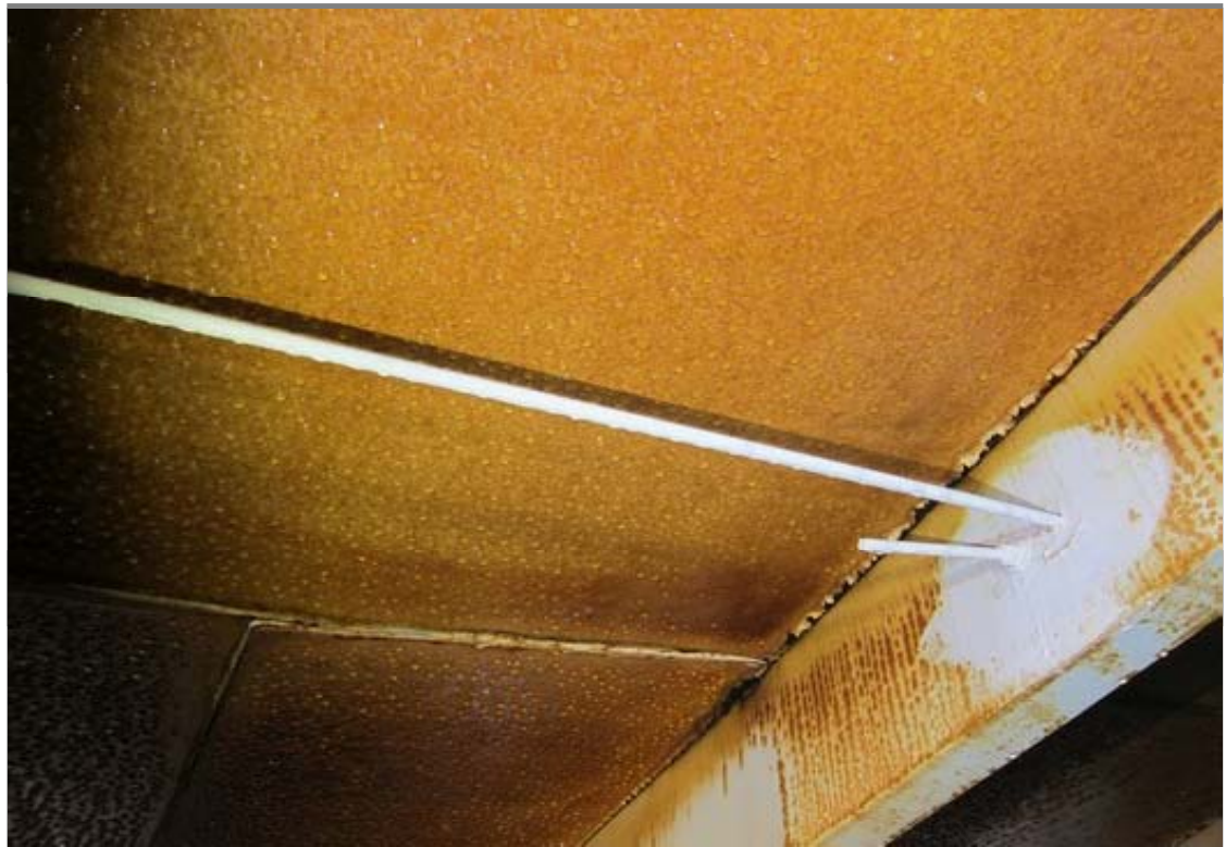
Additional view of the interior roof with rafter and bracing rods.
