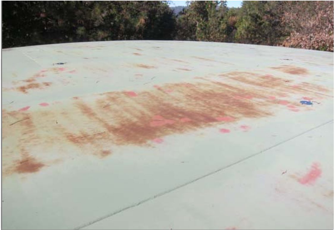
This view indicates the overall condition of the roof. The roof plate (steel) is in good condition but coatings are failing as indicated by the presence of general corrosion.
