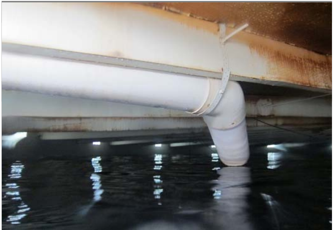
Interior view of inlet.
