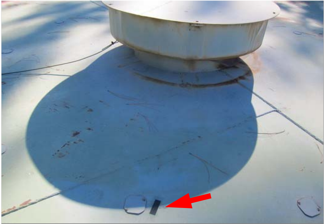
The roof vent consists of a steel cover over a steel riser pipe. The location identified by the arrow is a drilled hole that was temporarily sealed with tape by ATS, Inc.
