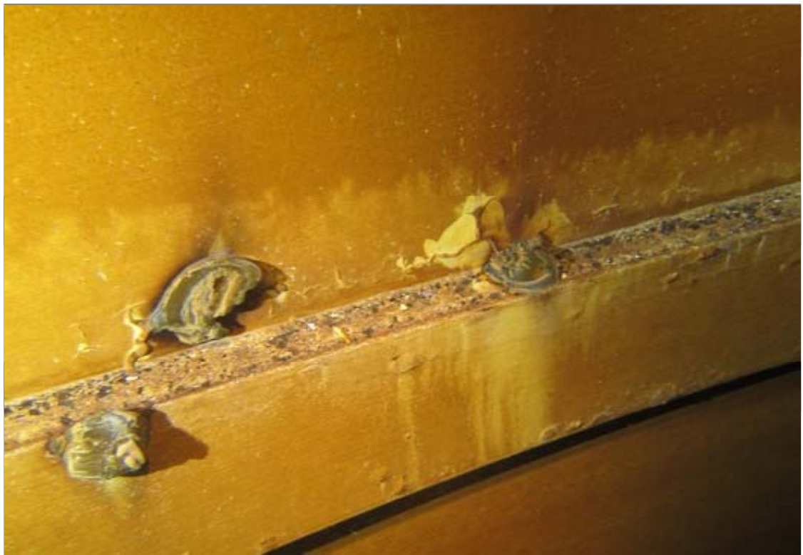
An additional view of corrosion nodules on the interior shell. The area shown is where a shell opening (door sheet) was cut and rewelded upon completion of the work. This area has a particularly high concentration of coating failures.
