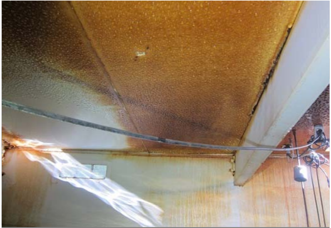
Upper shell and adjacent roof. Staining and general corrosion is present on most surfaces.
