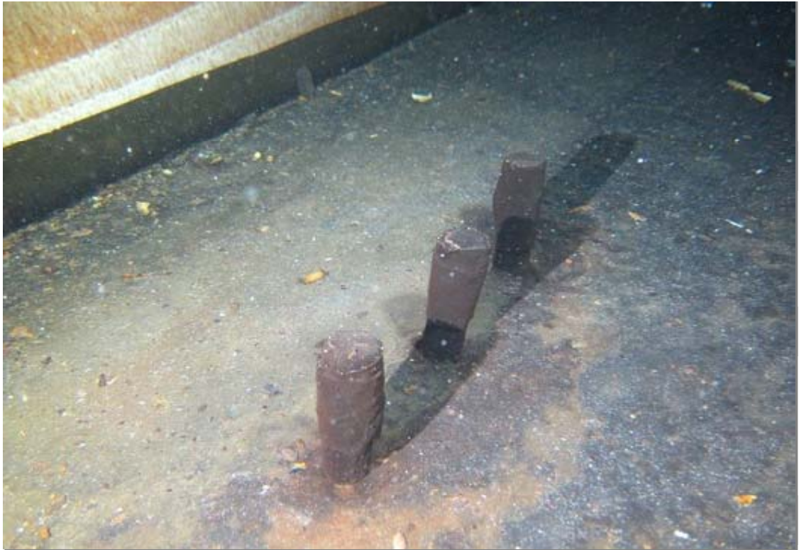
Unidentified pipes near the bottom penetrating outlet. These may be from an abandoned level gage.
