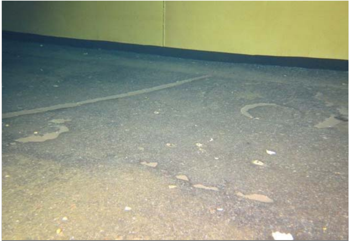
Lower shell and tank bottom. Coatings are in good condition overall in this zone.
